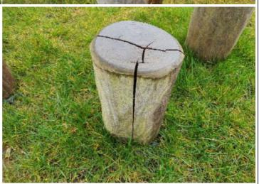
**Finding:** There are splits running through the timber that cross through or near fixing points and may cause instability in the future
