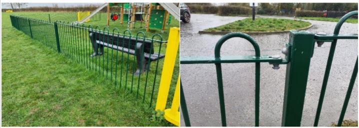
**Finding:** Shear nuts have not been fully tightened and are still present on fixings
