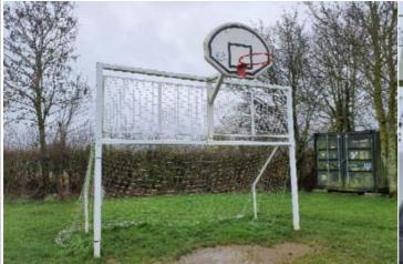
**Finding:** The item fails to meet the requirements of BS EN 15312 4.4.2.1 head and neck entrapment in the frame
