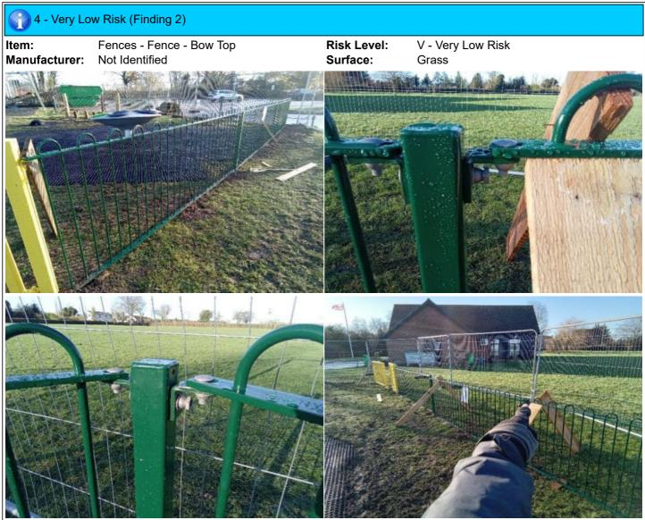
**Finding:** Shear nuts have not been fully tightened and are still present on fixings
